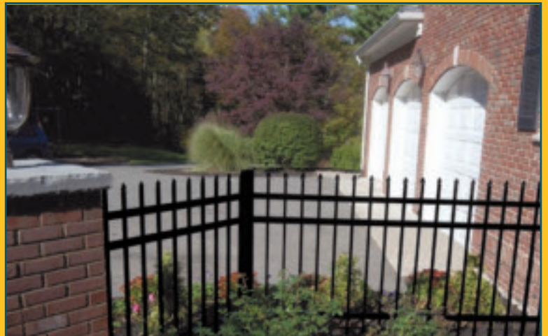
Three rail with pickets through top rail.
