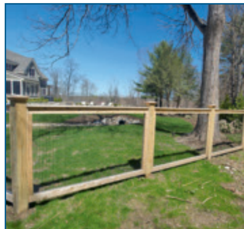
Wood-framed Welded Wire
